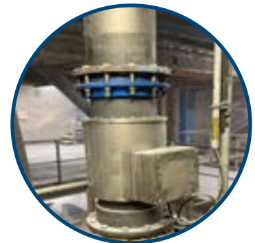
Coil with Measurement Board (Stainless Steel Housing)
