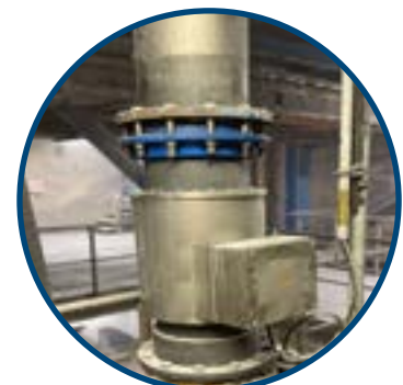
Coil with Measurement Board (Stainless Steel Housing)
