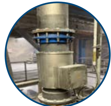
Coil with Measurement Board (Stainless Steel Housing)
